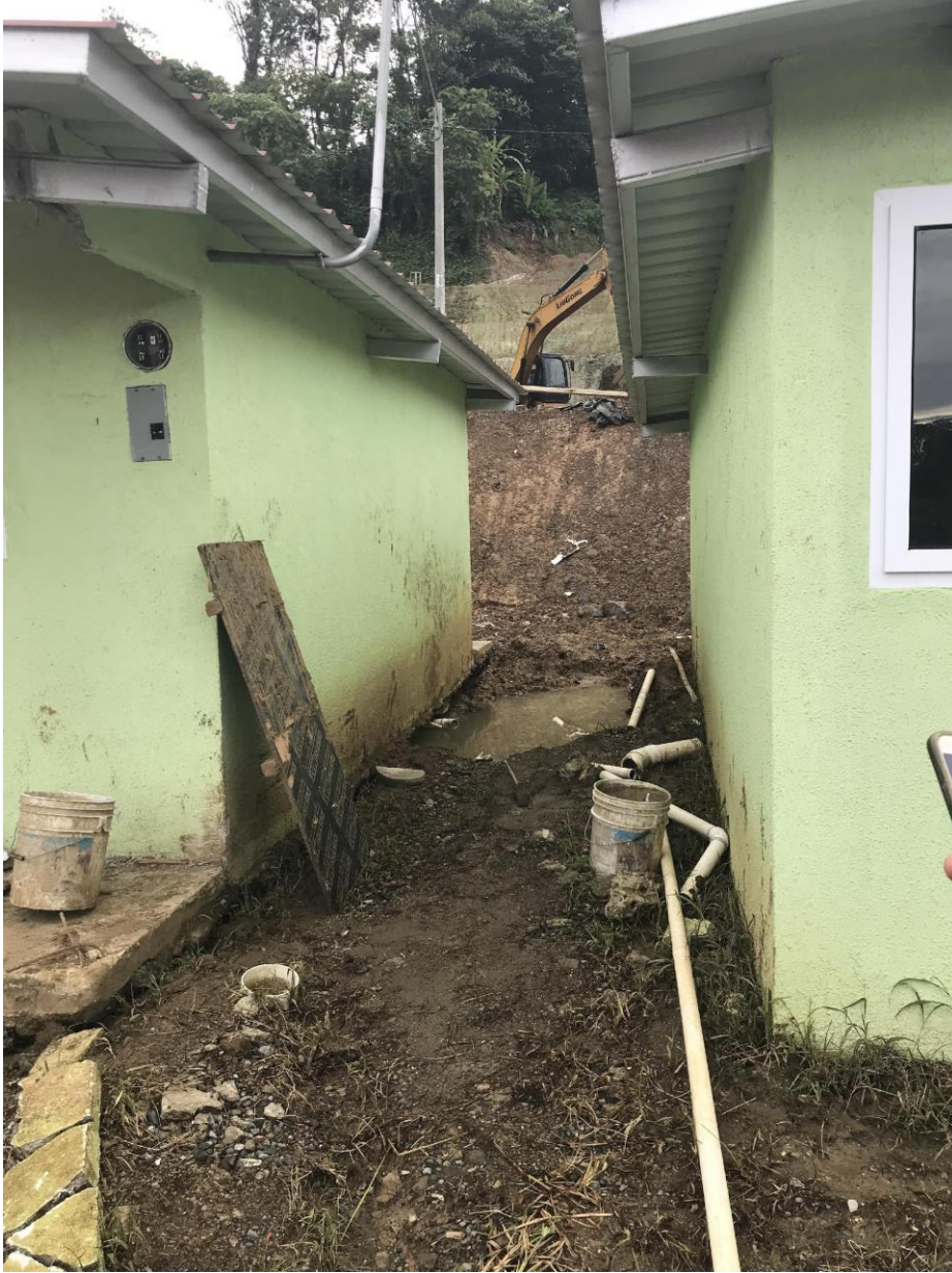
Figure 9 Image of water compiling at base of hill where houses are placed on top of wet soil without foundational support
