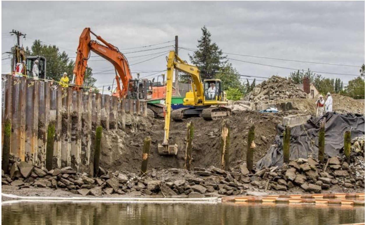
Figure 11. Restoration work by the Port of Seattle. A “conventional” restoration project in the LDR begins with regrading of the shoreline. ( “Lower Duwamish River Habitat Restoration Plan,” Port of Seattle )
